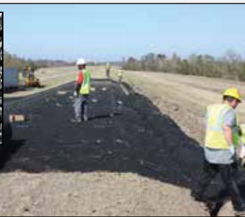
US Army Corps of Engineers Levee Construction
