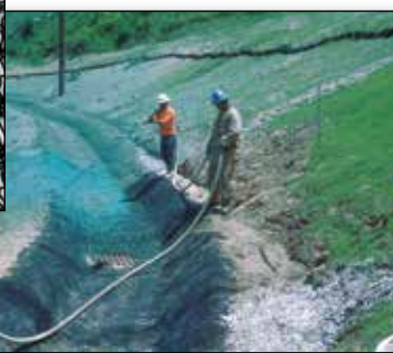
Slope interceptor ditch on steep slopes
