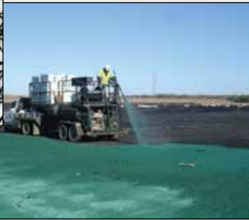
Flexterra® HP-FGM™ applied into TRM 7003
