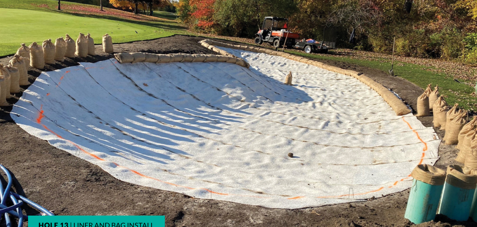
HOLE 13 | LINER AND BAG INSTALL
