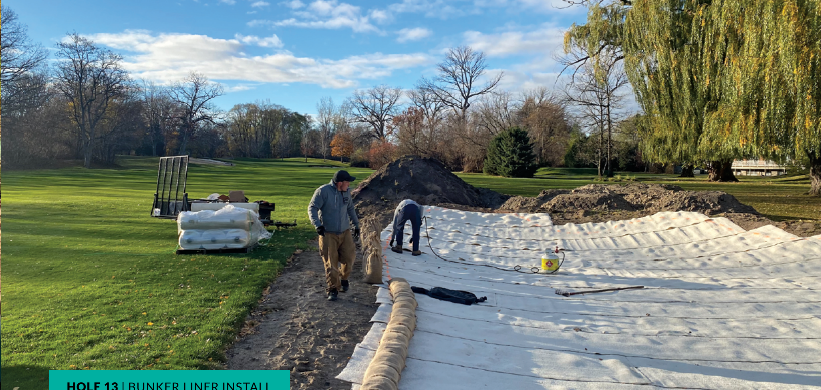
HOLE 13 | BUNKER LINER INSTALL
